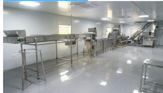
Figure 6: ABUAD's Existing Waste Recycling Plant
