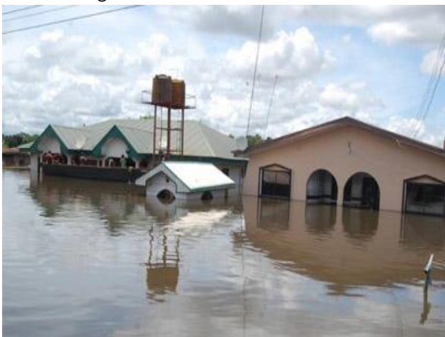
Figure 16.0: Flood affected residential buildings in Bayelsa State
