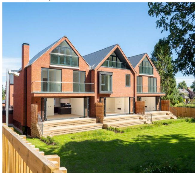
Figure 4.0: Flood-resistant homes that employ a host of innovative features to keep their residents dry have been built on a flood plain in Stratford-upon-Avon.
