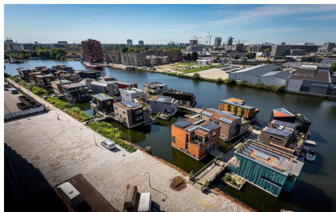
Figure 7.0: Floating homes development in Amsterdam.
