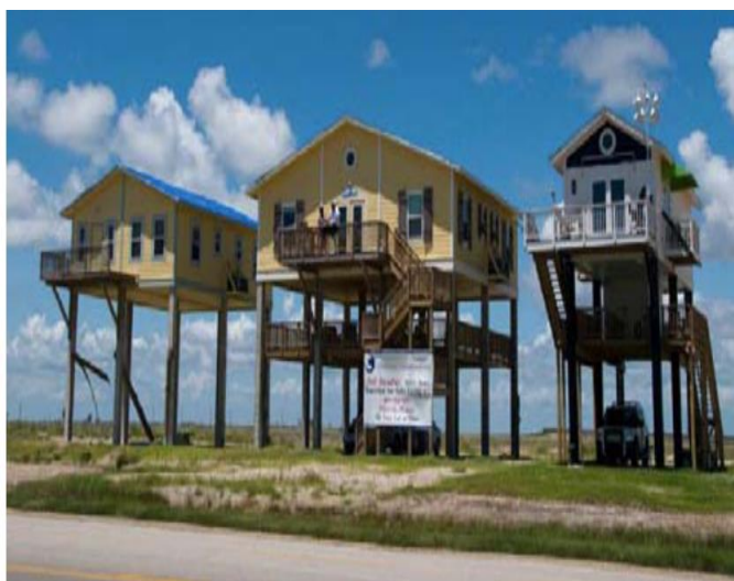
Figure 2.0: Elevated buildings in Galveston, Texas, United States of America
