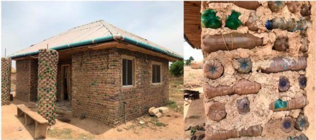
Figure 1. Waste bottle house in Paipe, Abuja, Nigeria. Source: Onyenokporo et al. (2024).
