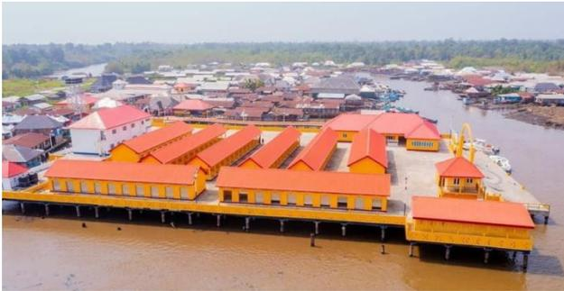
**Figure 28:** The Ogheye riverine community is close to the Ogheye Floating Market, Delta State. Note the sub-structural piers supporting the main deck of the market. Source: Authors' Fieldwork.
