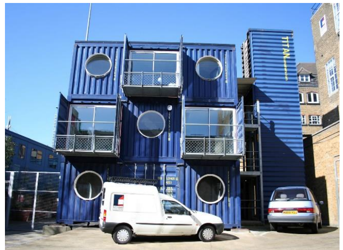
Fig 4.0: Image of the High School at the container City London, UK
