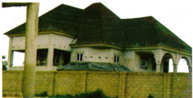
Plate 9, Contemporary compact rectangular house constructed of concrete blocks and corrugated roofing sheets.
