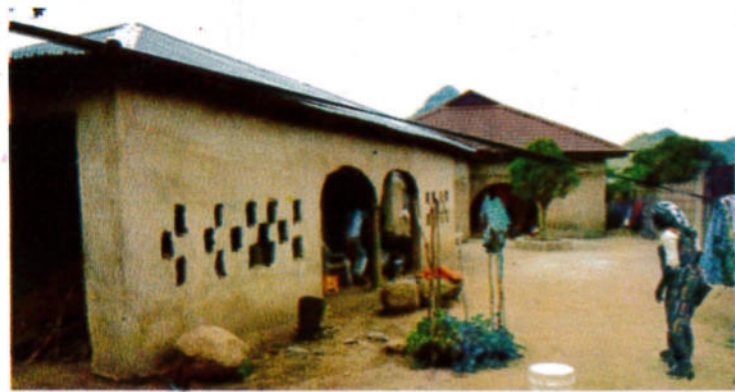
Plate 6 Contemporary house in Lapan, rectangular houses constructed of concrete and plastered with sand – cement mortar and corrugated Almunium roofing sheets.
