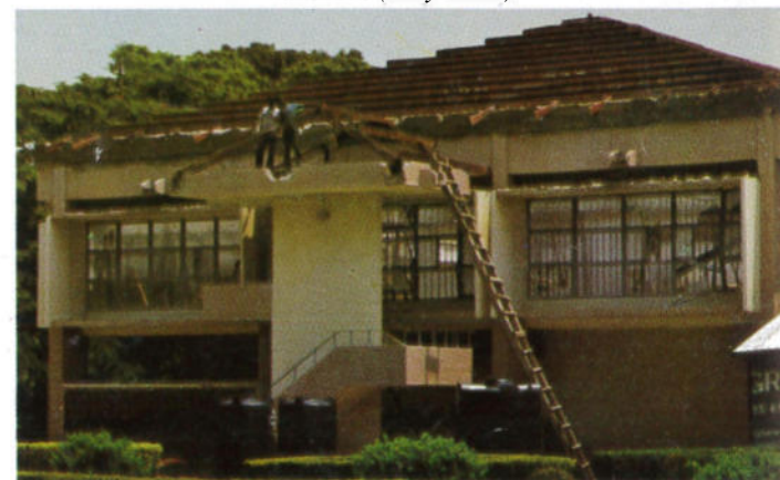
Plate 13. Lecture Theatre, Faculty of Pharmacy, Ahmadu Bello University, Zaria. Note the flat roof being replaced with pitched roof. Note also the spouts of the original roof gutter. Source: Photograph by the authors (July 2011).
