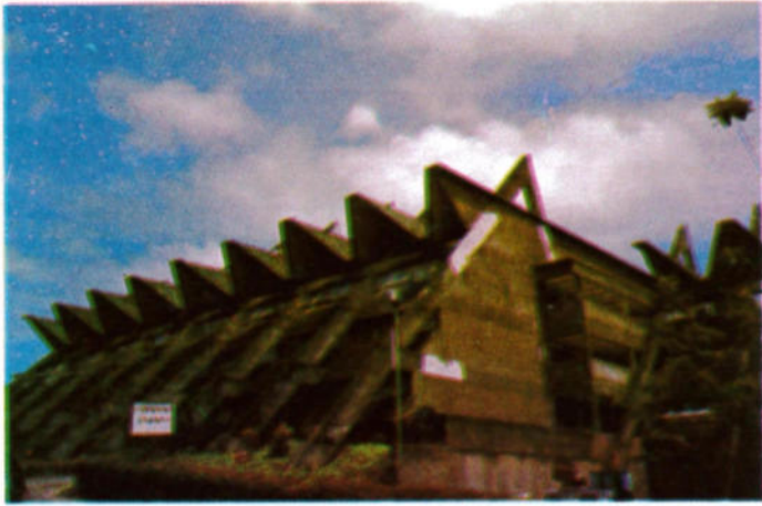
Plate 9. Department of Civil Engineering by Niger Consultants, Obafemi Awolowo University, Ile-Ife. Source: Photograph by the authors (October 2005).
