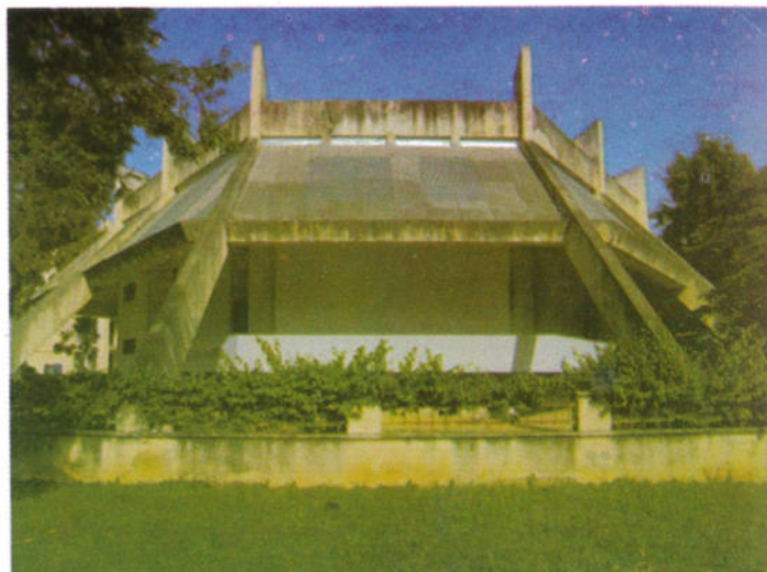
Plate 11. Umaru Shehu Lecture Theatre, aka Spider Lecture Theatre (Twin Lecture Theatre) by Niger Consultants, Ahmadu Bello University, Zaria. The sloping roof slabs were covered with felt and drained into concrete gutters. Source: Photograph by the authors (September 2005).
