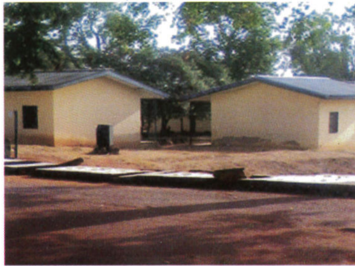
Plate iv: Front View Village Hostel Compound 8
