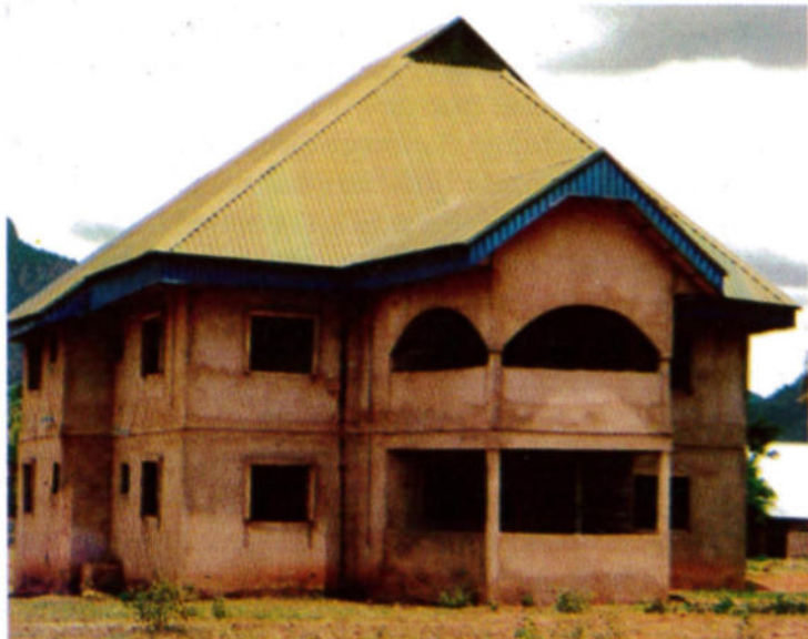
Plate 10, Contemporary compact rectangular house constructed of concrete blocks and corrugated roofing sheets.
