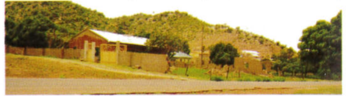
Plate 4 Contemporary house in Lapan, a four bedroom bungalow constructed of concrete blocks and corrugated galvanized iron roofing sheets.
