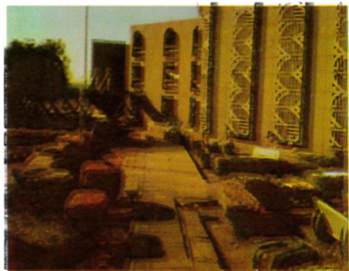
Front View Abuja Hostel Block D
