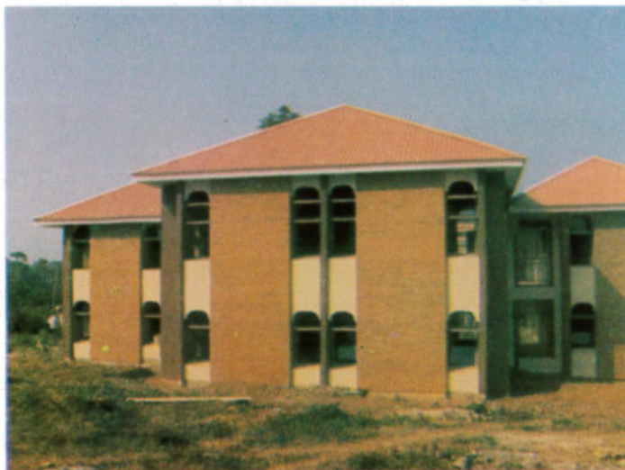
Plate 15. School of Earth and Mineral Sciences by Soft Designs Environmental Consultants Ltd (2004), Federal University of Technology, Akure. Note the use of brick facing and recessed openings and walls. Source: Photograph by the authors (December 2006).
