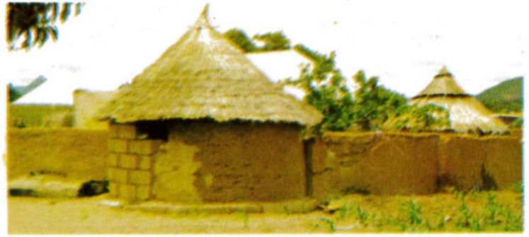
Plate 2c. A compound with combination of traditional cylindrical house form with thatched roof and rectangular house form in the background with corrugated galvanized iron hip roof
