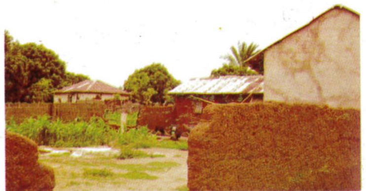
Plate 5 Contemporary house in Lapan, rectangular houses constructed of mud and plastered with sand - cement mortar and corrugated galvanized iron roofing sheets.
